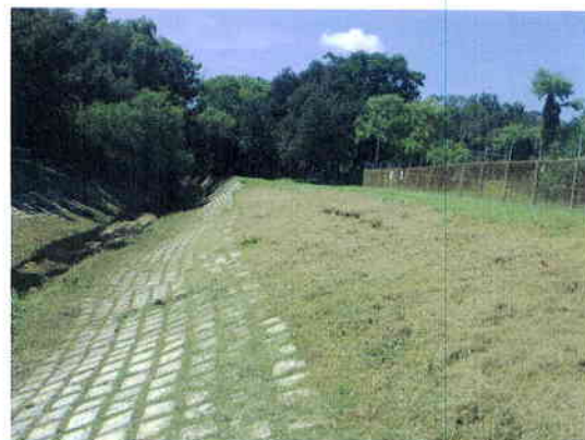
Channel 4 looking west
