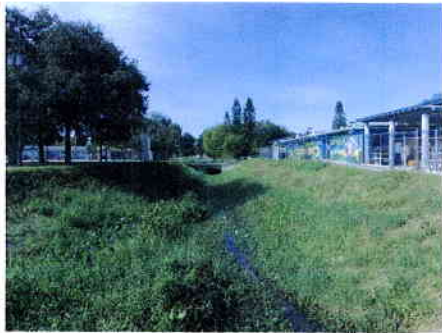
Channel 1AW west of pedestrian bridge
