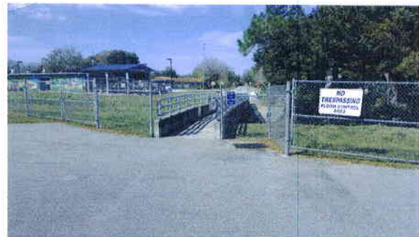
Pedestrian bridge crossing Channel 1AW
