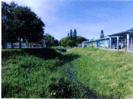
Channel 1AW west of pedestrian bridge
