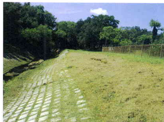
Channel 4 looking west
