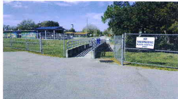
Pedestrian bridge crossing Channel 1AW
