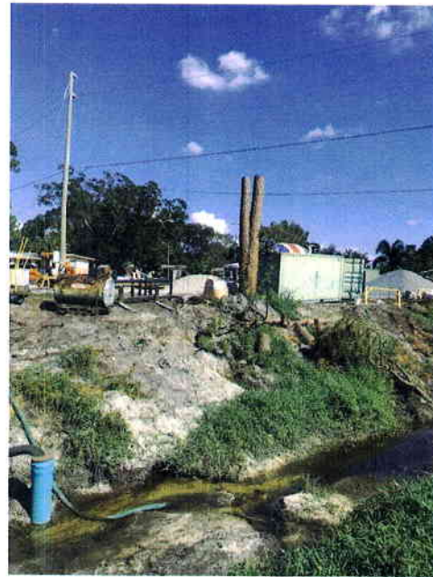
Channel 1AW east of pedestrian bridge
