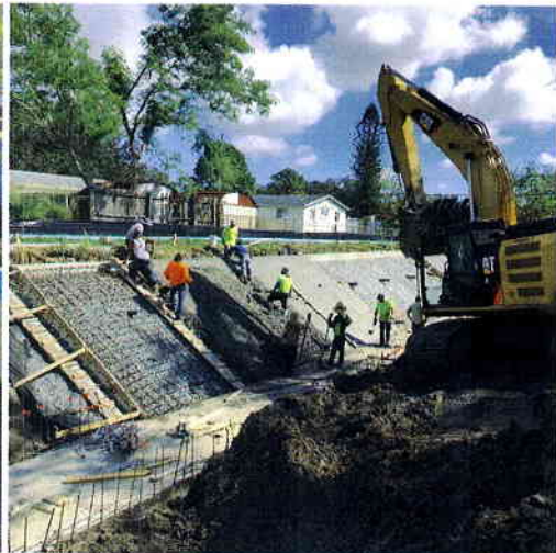
Pouring north bank
