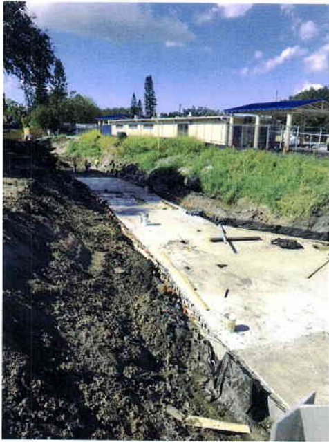
Channel 1AW west of pedestrian bridge
