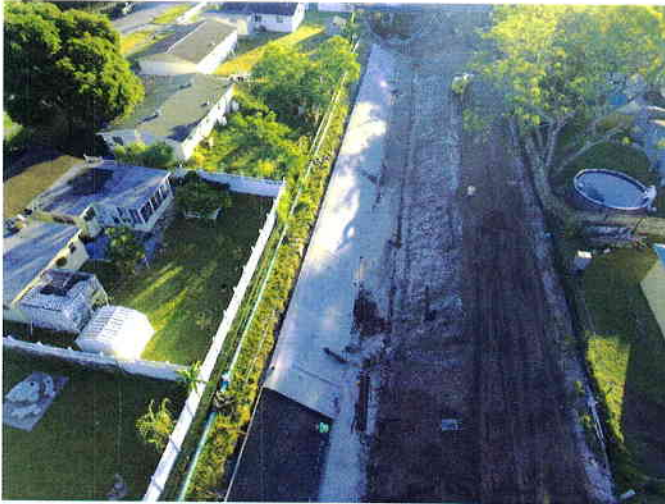
Channel 1AW west of 58 th Street
