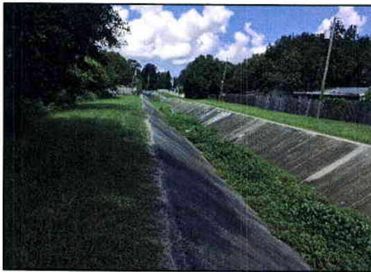
Channel 1B5 – Looking west along Channel 1B5
