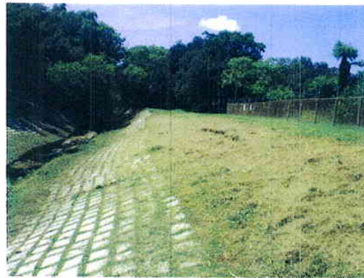
Channel 4 looking west
