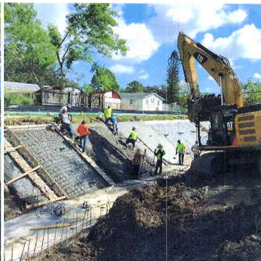
Pouring north bank
