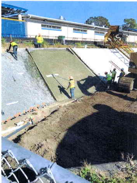
Ch 1AW north bank west of ped bridge
