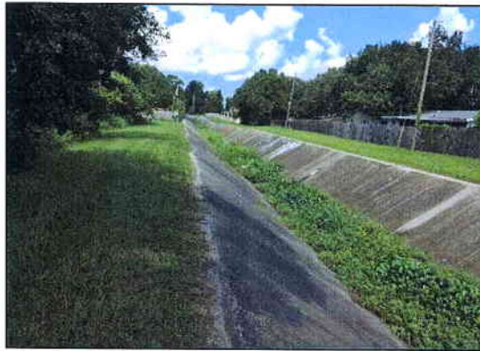
Channel 1B5 – Looking west along Channel 1B5
