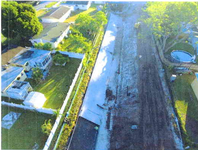
Channel 1AW west of 58 th Street
