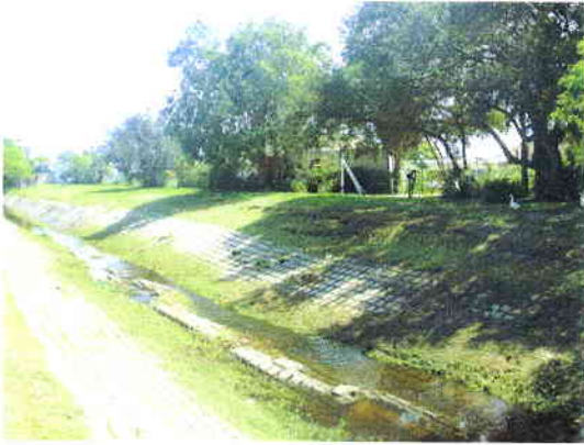
Channel 4 looking east
