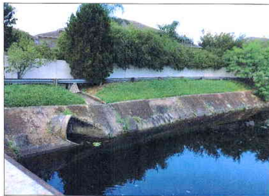
Channel 1 – Looking southwest from 66th Street
