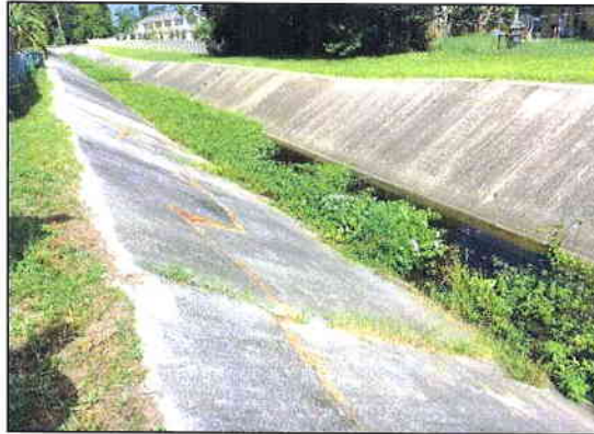
Channel 1B5 – Looking west along Channel 1B5 near 59th Street
