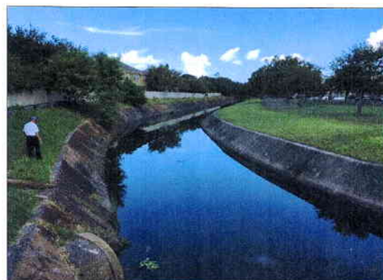
Channel 1 – Looking southwest from 66th Street
